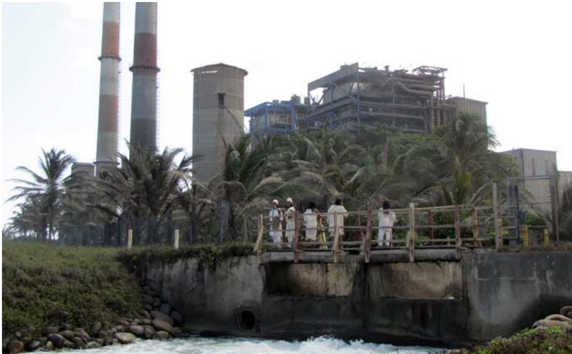
Power plant at the sacred site of Compañía.
